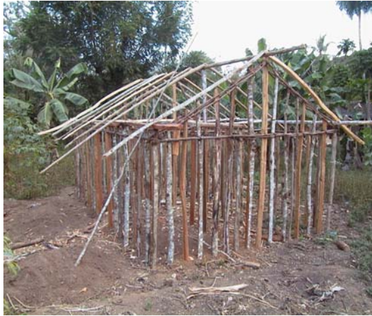
Figure 7 Evidence of use of indigenous trees for construction poles (Field photo, 2006)
